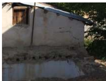
Figure 3. Corner failure in the presence of unconnected intersecting walls
