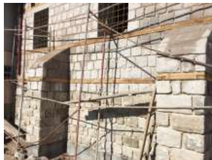
Figure 6. Re-pointing strengthening method
