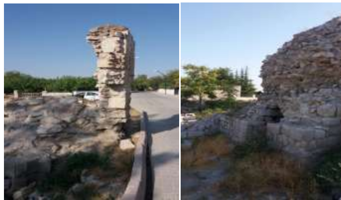
Figure 2. Out-of-plane collapse
