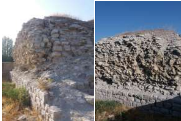
Figure 4. Stone dislocations and collapse
