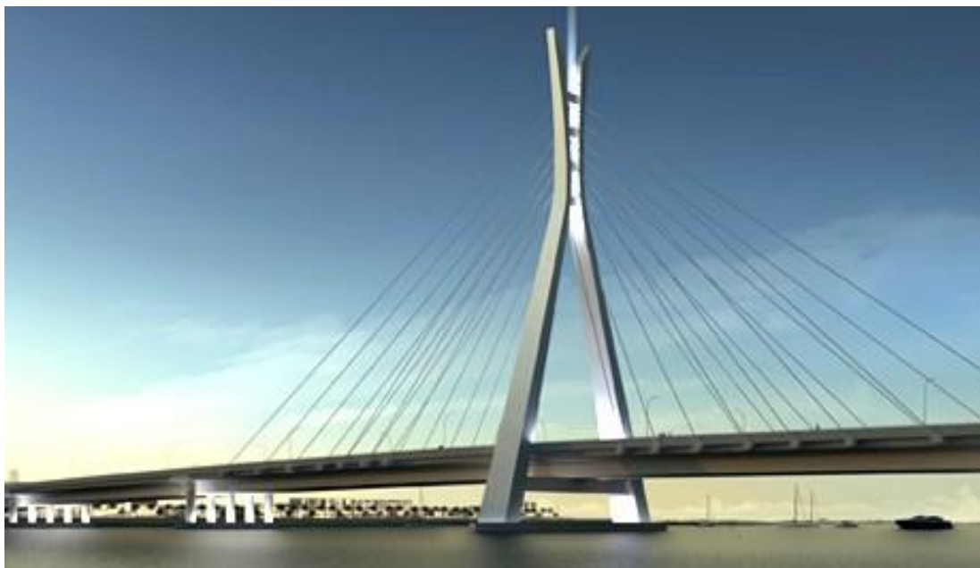
Figure 3.1: Lekki cable stayed bridge (Julious Berger Plc, 2013)
