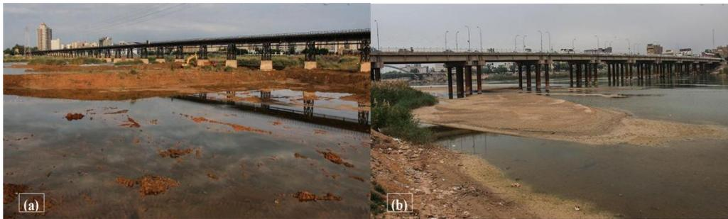
**Figure 20:** View of the islands formed by the river sedimentation at the downstream;
