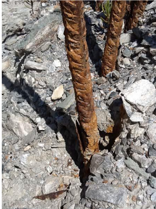
Photo 1: Corroded reinforcements.
