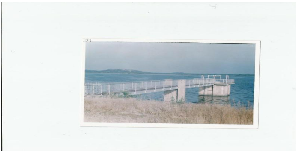
Figure 4: View of Gubi dam water intake point
