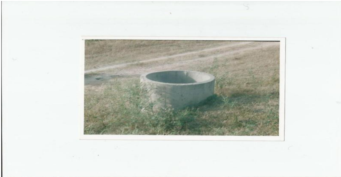
Figure3: View of control well in Gubi dam treatment plant
