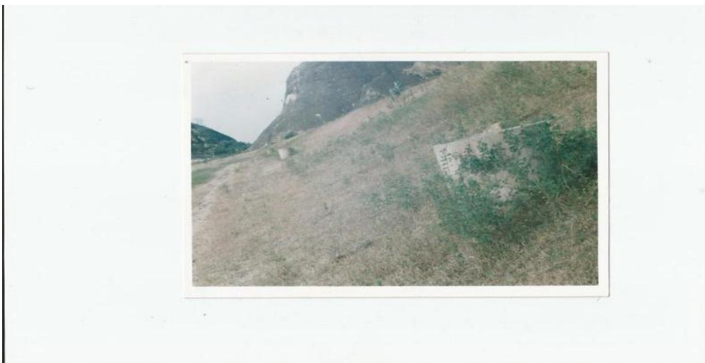
Figure 5: View of Embankment of Gubi dam
