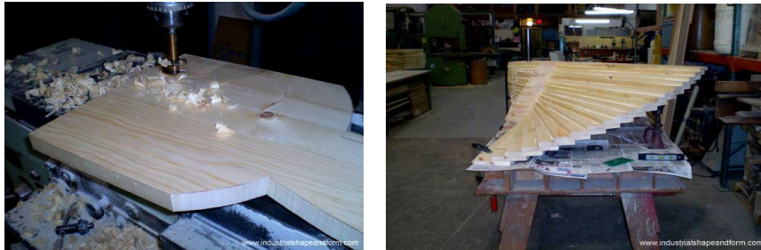
Figure 2. Center hole drilling and stack of offset wood layers
