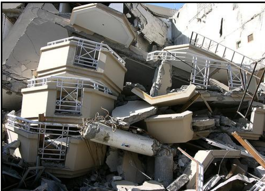
A total collapse of a building
