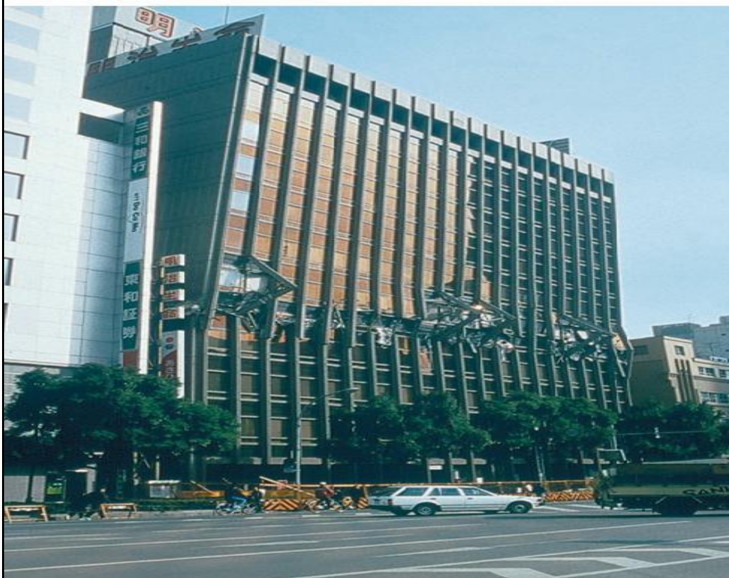
Sway mechanisms are often inevitable with soft storey ground floors (Izmit, Turkey 1999)
