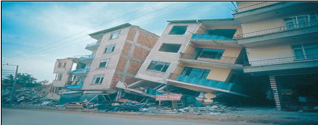
Sway mechanisms are often inevitable with soft storey ground floors (Izmit, Turkey 1999)
