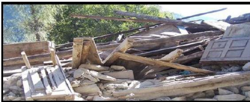
Stage IV of Earthquake. Damage
