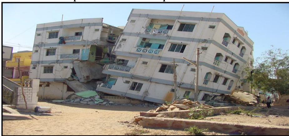
Collapsing a building
