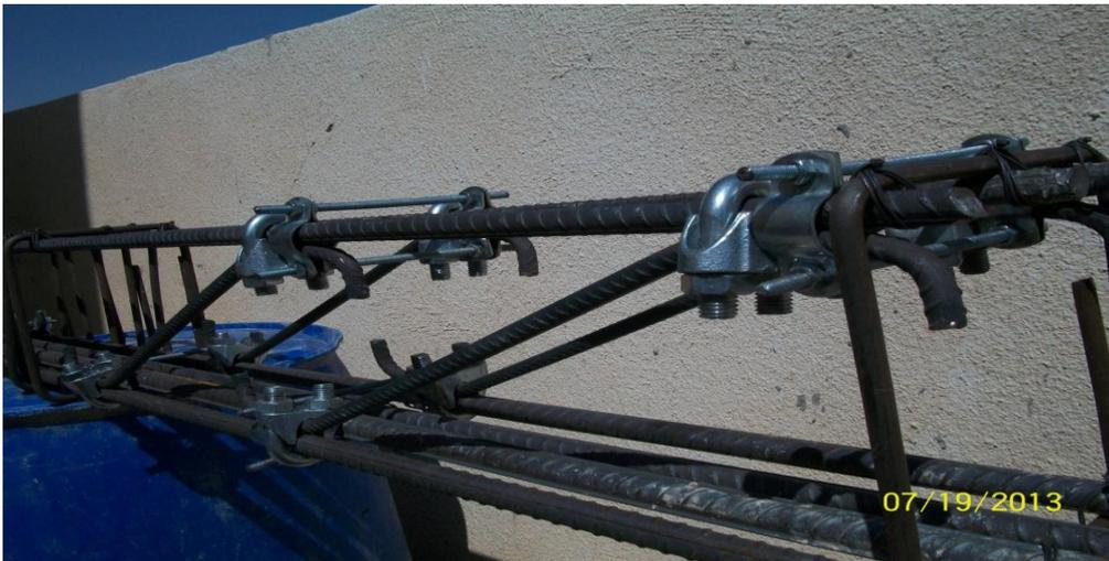
Figure 3: Steel cage reinforcement of beam BB bolted swimmer bars.
