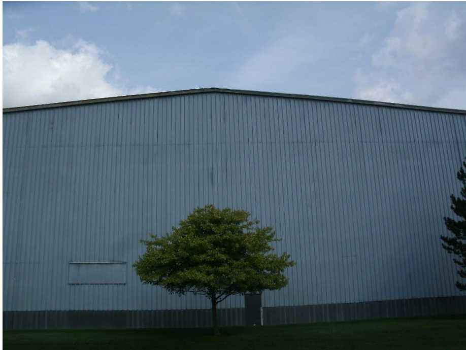
Fig.1. Structure with a Gable Roof. (Author photo.)
