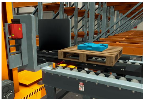
Figure 11. Stacker crane – forks carry
