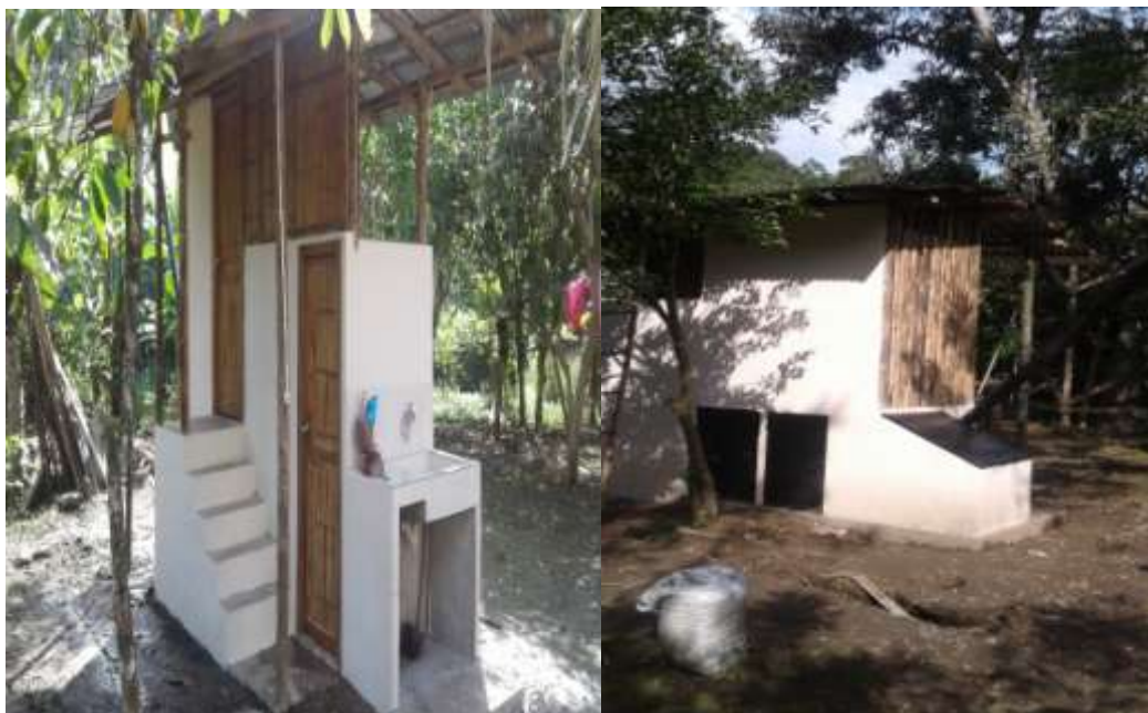
A WASH unit installed in a rural community, Junín, Ecuador. Photo: Bruno Bellettini.
