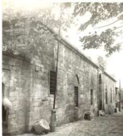
Photo 9. The facade of the madrasa from the Haseki Street (Archives of Directorate of Foundations, repair records, 1960)
