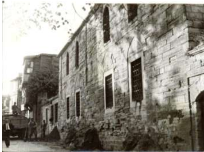
Photo 12. Facade of the school on the Haseki Street (Archives of Directorate of Foundations, repair records, 1967)
