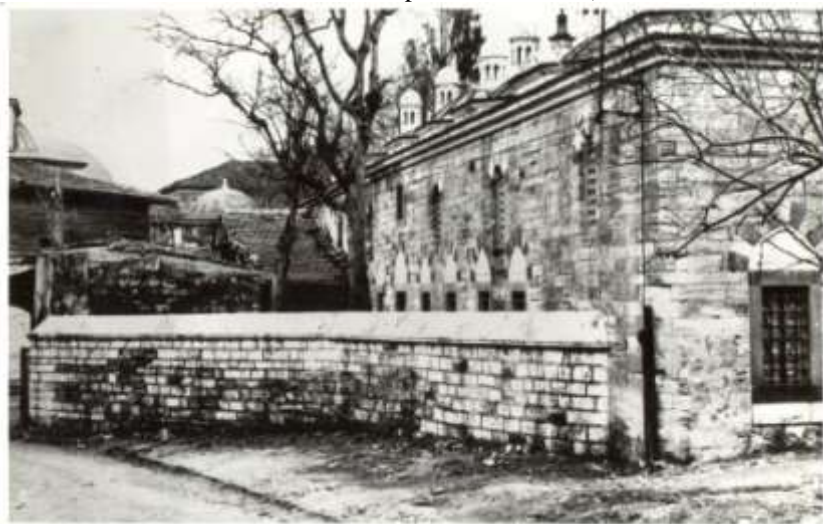
Photo 11. Facade of the madrasa towards the Sami Paşa Street, after restoration (Archives of Directorate of Foundations, repair records, 1960)
