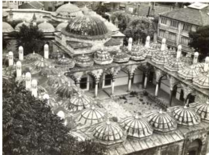
Photo 8. The Haseki Madrasa (Archives of Directorate of Foundations, repair records, 1964)
