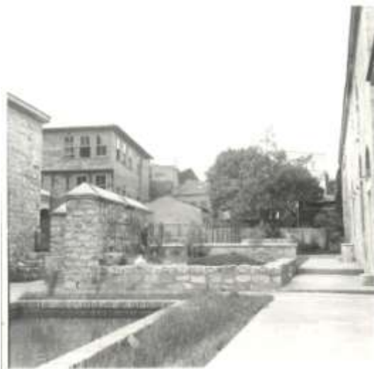
Photo 20. Haseki İmaret (Kitchen) and the wooden houses (Archives of Directorate of Foundations, repair records, 1968)
