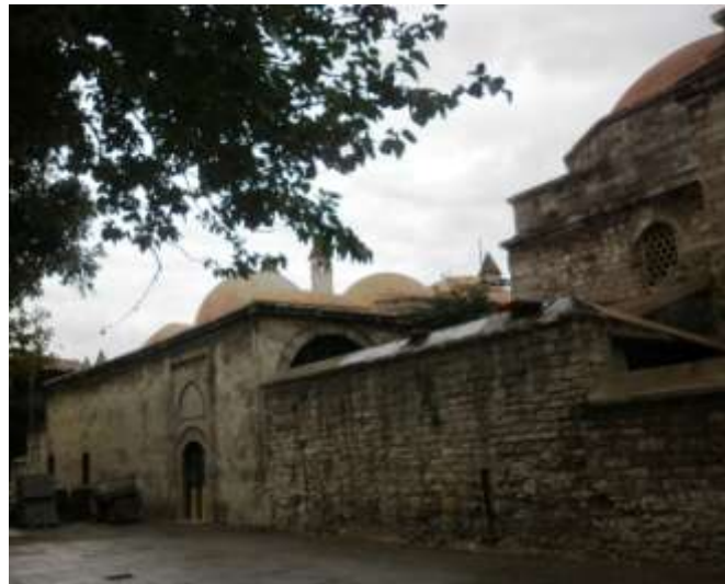
Photo 22. North facade of the Haseki Darüşşifa (Hospital) (2010)
