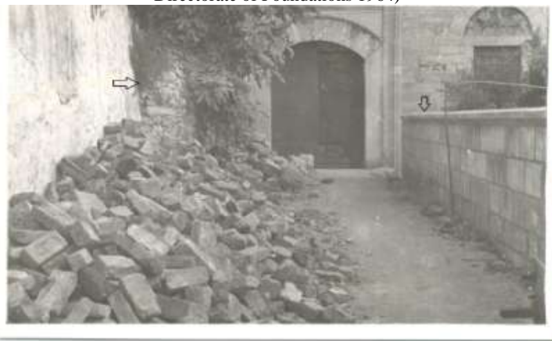
Photo 16. İmaret Aralığı (Kitchen Passage) (Archives of Directorate of Foundations, repair records, 1964)
