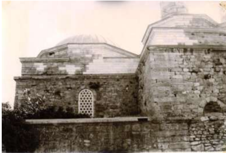
Photo 14. The fountain storage and the kitchen (Archives of Directorate of Foundations, repair records, 1964)
