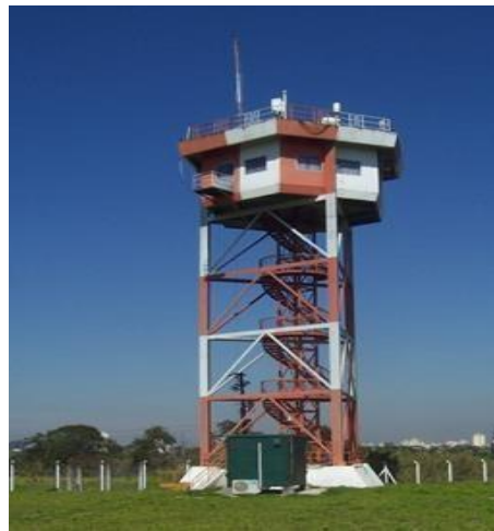
Fig.01. ACA tower at 25 m above ground
