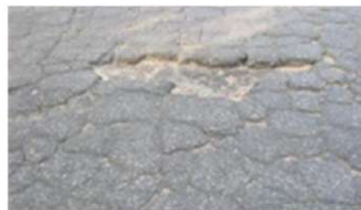
Plate 2: Fatigue Cracking
