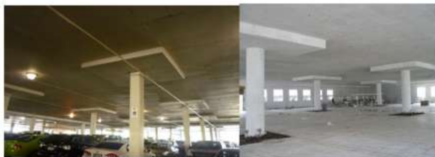
Fig. 1.1: Flat slabs with Drop Panels
