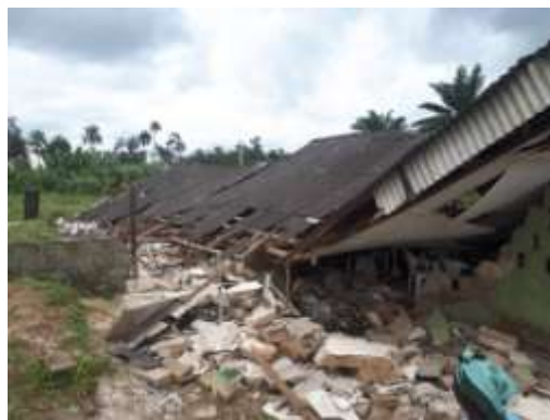
Figure 2. showing a cross section of collapsed St. Paul's Catholic Church at Adagrassa-Ugolo, Okpe LG.A., Delta State, Nigeria on 2 nd September, 2018. Source: Bldr. Kingsley Oghoro picture coverage.
