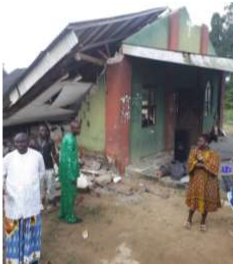
Figure 1. showing the front side of collapsed St. Paul's Catholic Church at Adagrassa-Ugolo, Okpe LG.A., Delta State, Nigeria on 2 nd September, 2018. Source: Bldr. Kingsley Oghoro picture coverage.
