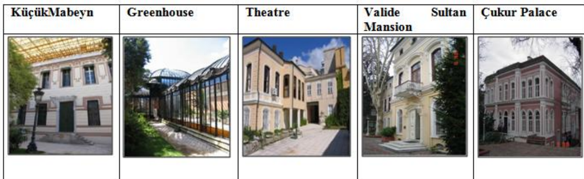
Fig. 4. Buildings located in second courtyard(AliasghariKhabbazi, 2016)
