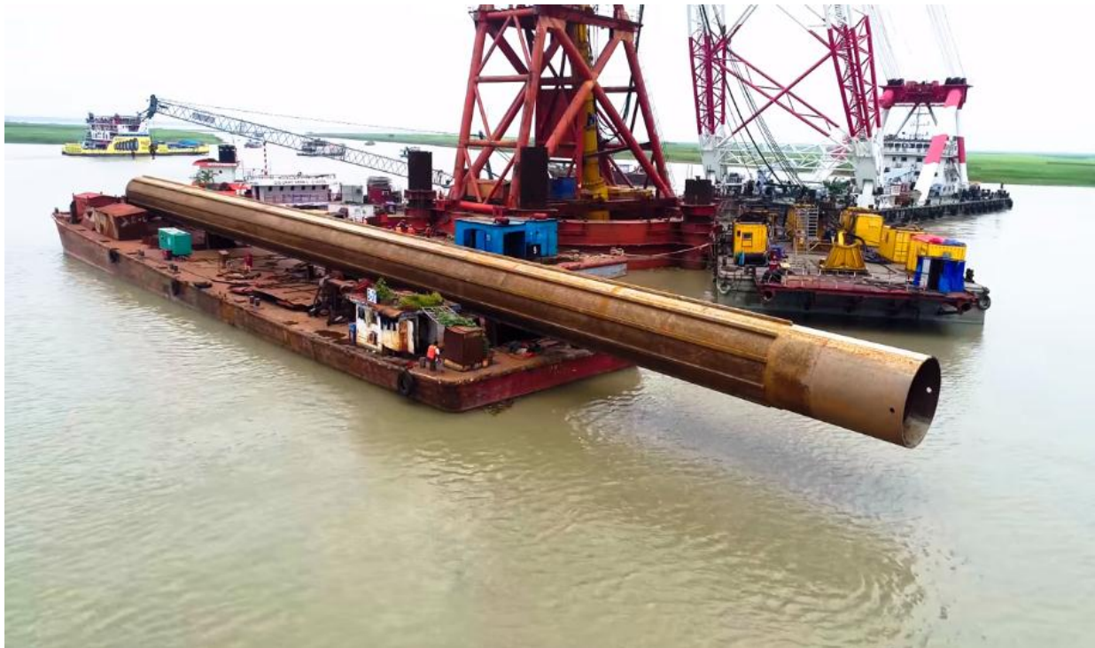
Figure 6: One Segment of steel tubular pile manufactured in Piling Yard
