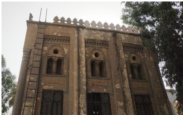
Image (50 ) shows Completing the installation of the missing sharrafat Eastern facade
