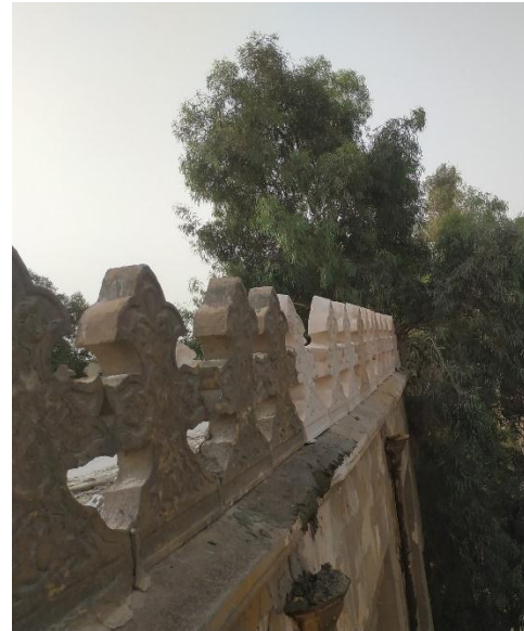
Image ( 49) shows Completing the installation of the missing sharrafat Eastern facade
