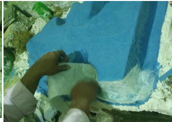
Image (17 ) shows Reinforcement with fiberglass
