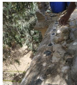
Image ( 33 ) shows Fill cement mortar around the coils to fix them
