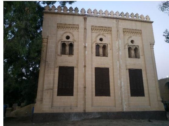
Image (51 ) shows Completing the installation of the missing sharrafat Western facade
