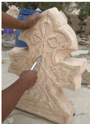
Image (38 ) shows Dividing one of the sharrafat to create a corner piece
