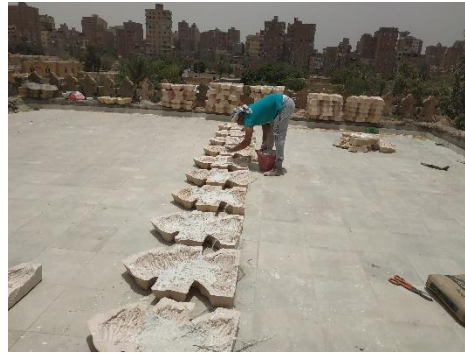
Image (36 ) shows Making linen bands at the back of each sharrafa
