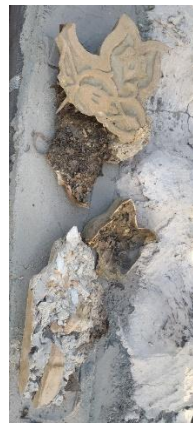
Image (4) shows the formations of artificial stone (sharrafat) and shows the empty core with Sawdust and is considered a hollow cast. There is another part with solid casting and stone fragments
