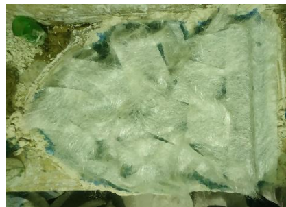
Image (20 ) shows Re-reinforcement with a second layer of fibers
