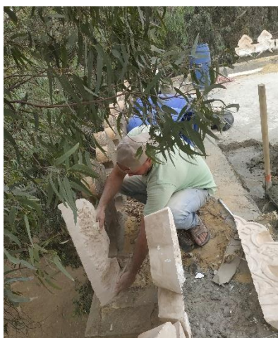
Image (45 ) shows Installing the corner piece
