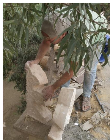
Image (46) shows Installing the corner piece
