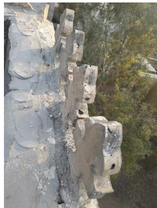
Image (3) shows the formations of artificial stone (sharrafat) and shows the holes that confirm that the core is empty and is considered a hollow cast.
