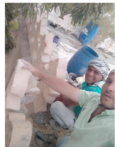
Image (47) shows Installing the corner piece
