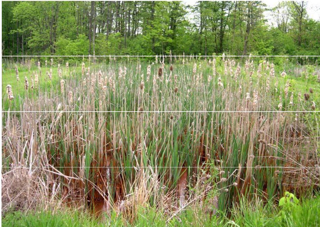
Figure 5. A FWS CW for tertiary treatment of municipal wastewater in McGrath Hill, Hawkesbury, near Sydney, NSW, Australia. Photograph taken by the author.
