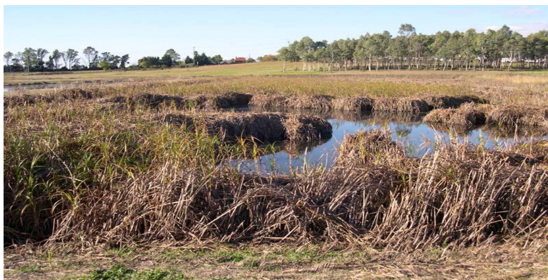
Figure 5. A FWS CW for tertiary treatment of municipal wastewater in McGrath Hill, Hawkesbury, near Sydney, NSW, Australia. Photograph taken by the author.
