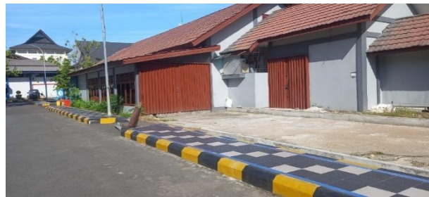
Figure 4. Sidewalk segment E (above) and F (bottom) in Polnep campus shows no shading system applied
