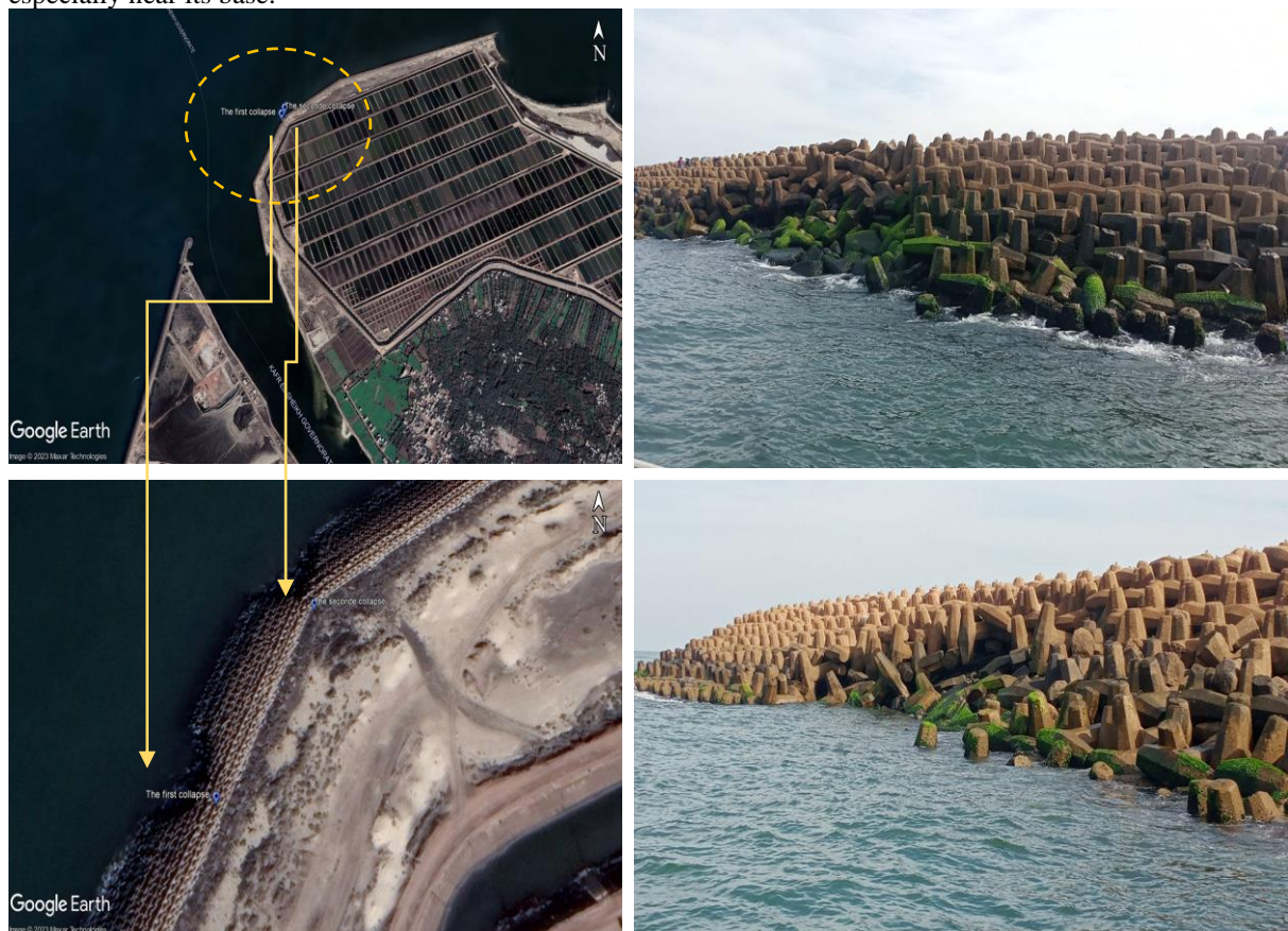
Figure 23. The last deterioration of the Rosetta Eastern Sea wall occurred in 2022.
