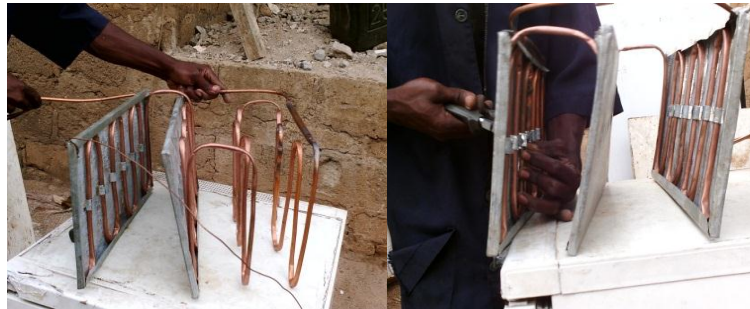
Plate 2: Evaporator Coil laid under its tray with 9 inches spacing
