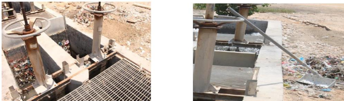
Fig. 3.3 The work of the filters and the tool used to filter the filters from sus. materials.
