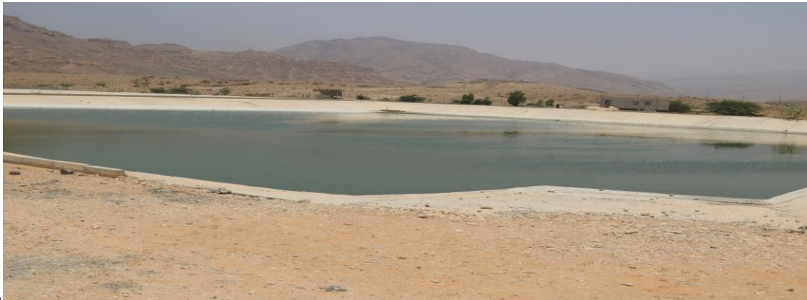
Fig. 3.4 A picture of anaerobic ponds
