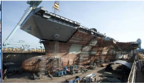
Painting and Pre-Erection
