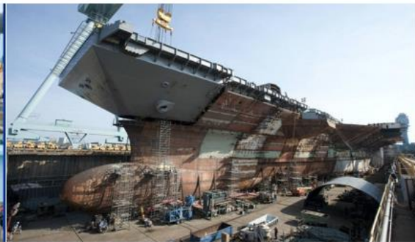
Painting and Pre-Erection
