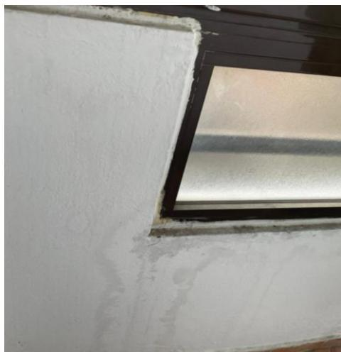
**Fig.17 Visible moisture on the wall, Building A**
