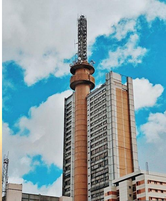
Fig. 2: NECOM House, Lagos [13]
