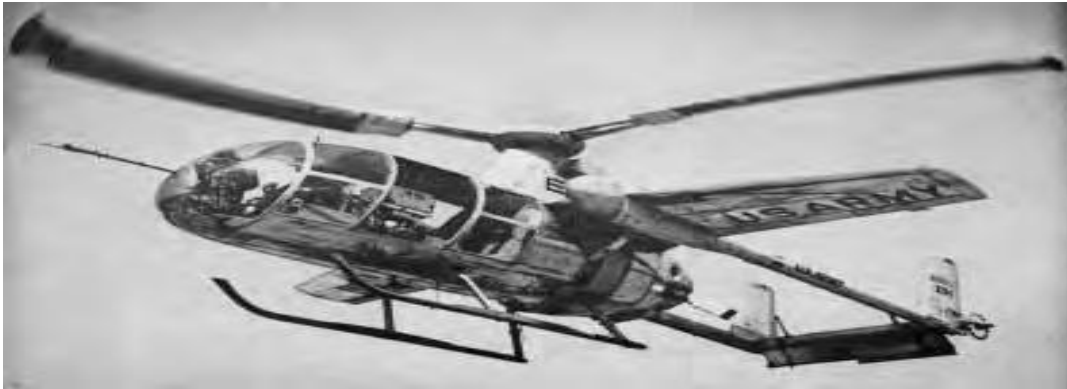
Figure 2. McDonnell XV-1 compound helicopter(Boeing Fotoğraf AD98-0209-13).
