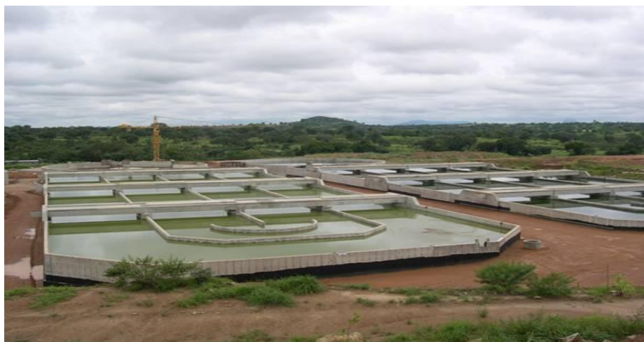
Figure 2.3: Shows the second part of Wupa Wastewater Treatment Plant
