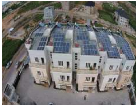
Figure 2: Solar-Wind Hybrid mini-grid systems with solar water heating systems at Guzape, Abuja. Holistic retrofits can achieve 50-90% final energy savings in thermal energy use in existing building with the cost savings typically exceeding investments.
