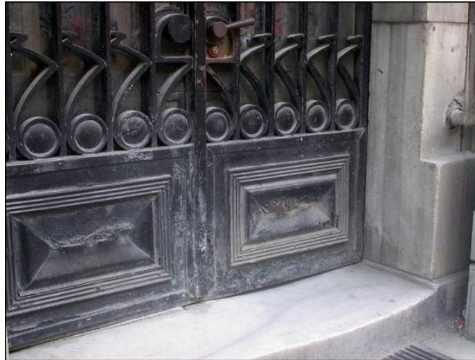
Figure 3. Deflection and material loss occurred by reason of usage at marble step (S.O.Hattap)
