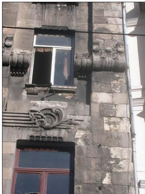
Figure 4. Occurrence of disintegration-surface erosion on the material by combination of mineralogical structure of Stone Material and some deterioration mechanisms in rain water such as acids and salts (S.O.Hattap)
