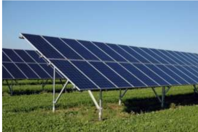
Figure 3: Solar PV array
