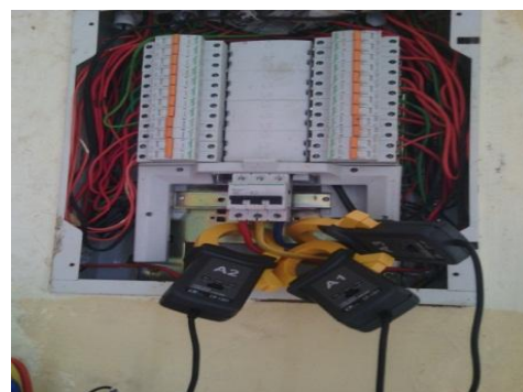
Fig 2: Power& Harmonic Analyser(DW6095). Fig. 3: Connection of probes at PCC
