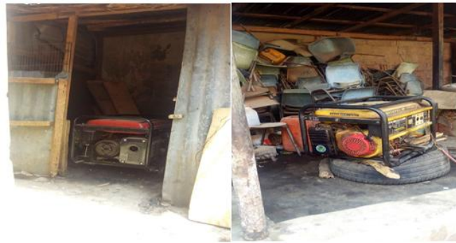
Plate 2: House-Keeping Practice of Generators in Residential Buildings in the Transition Zone
