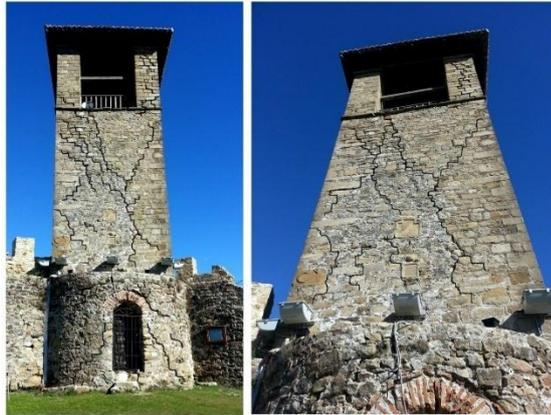
Figure 4. Structural cracks found on the main façade.
