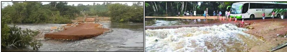
Figure 14. A. Rio Arataú damages bridge and passengers expect the transport service re-establishment. Source: Diário do Pará, 2014.
