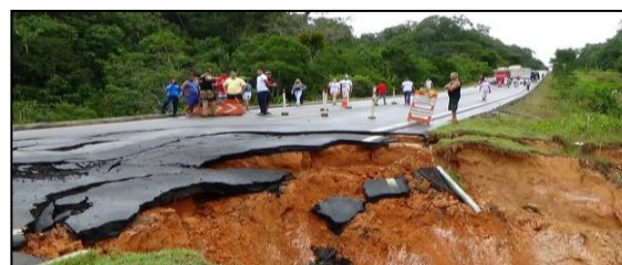
Figure 4. BR-174. Disruption by erosion. 117 km from Manaus. Source: G1 Amazonas, 2014.
