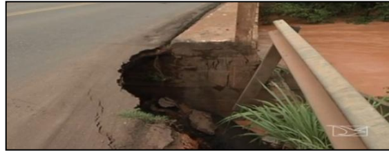
Figure 13. A. damaged bridge on US-010. Source: G1 Maranhão, 2014.
