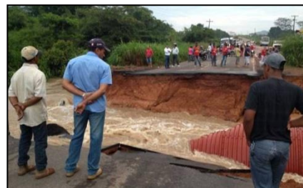
Figure 12. Culvert collapsed on the BR-155. Source: G1 Pará, 2014.
