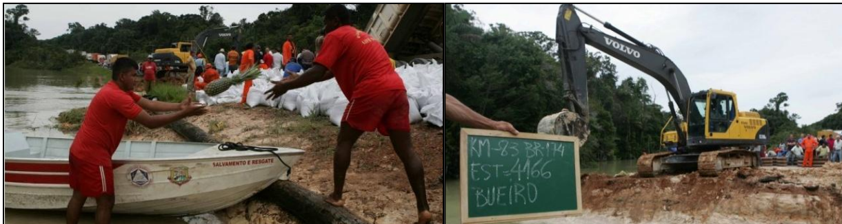
Figure 5. Disrupt in BR-174 by pipe rupture gallery. Source: D24AM, 2011.
