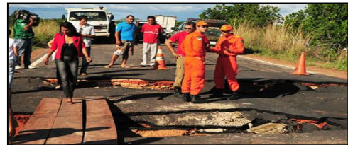
Figure 9. Drain tubes Break in the BR-401 highway. Source: A Critica, 2012.
