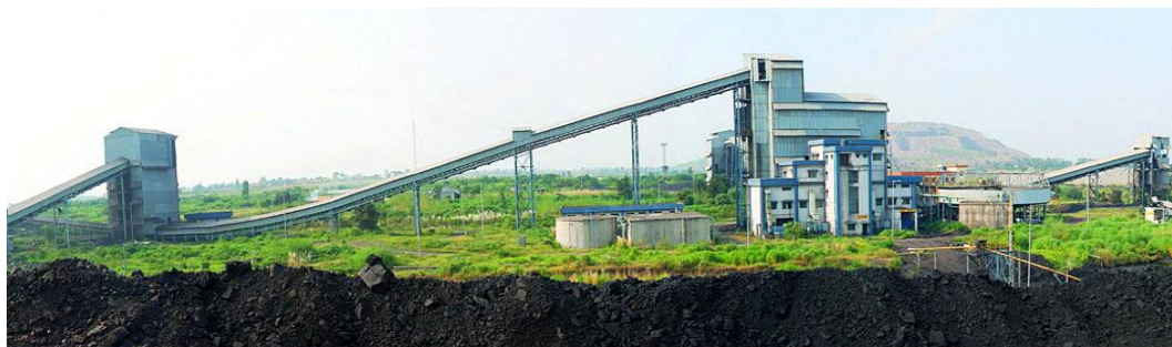
Fig. 1 View of Bhojudih Coal Washery under (BCCL)
