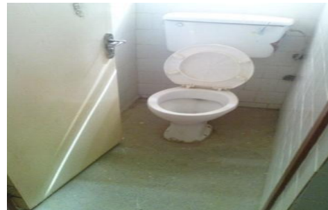
(b) F.U.T staff school (staff toilet )no consideration for door swing (Problem for wheel chair users)
