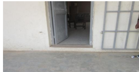
(B) F.G.C Minna: door width to offices Are too small and threshold Presence In Doorways Prohibits Easy access To Disabled Users
