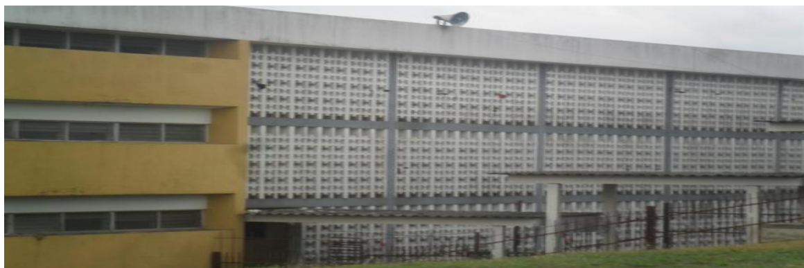
Fig. 1: General view of the case study building (a) roof overhang (b) screen wall
