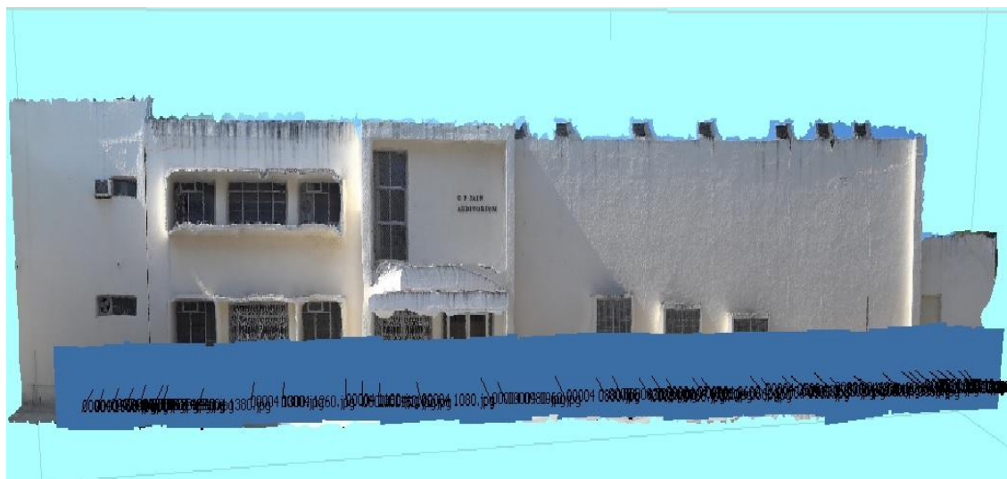
Figure 5. Building façade with video frame positions
