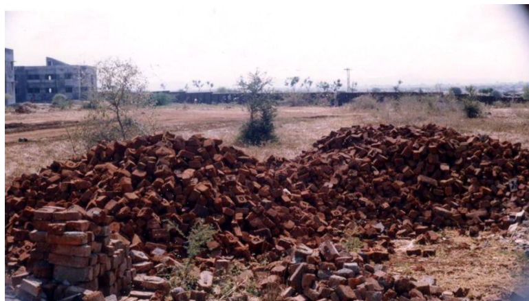
Fig 2 Improper stackig of brick
