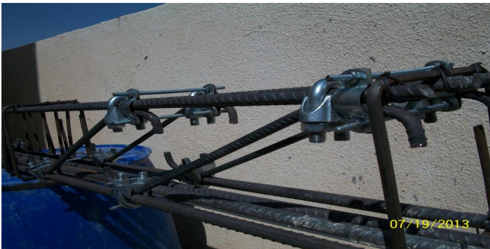
Figure 3: Steel cage reinforcement of beam BB bolted swimmer bars.
