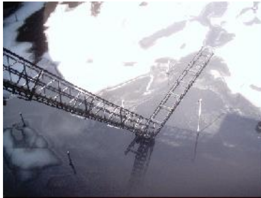
Figure 2: FRT Roof Access Ladder
