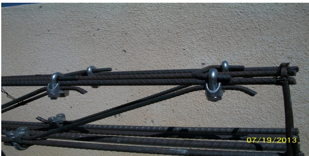
Figure 4: Steel cage reinforcement of the beam, BU, U-link bolted swimmer bars.
