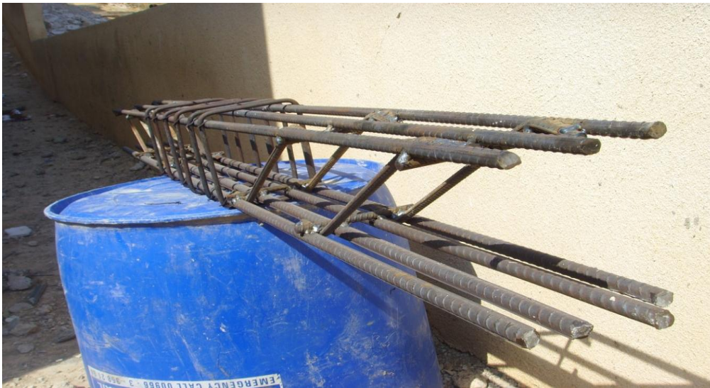
Figure 2: Steel cage reinforcement of the beam BW, welded swimmer bars.
