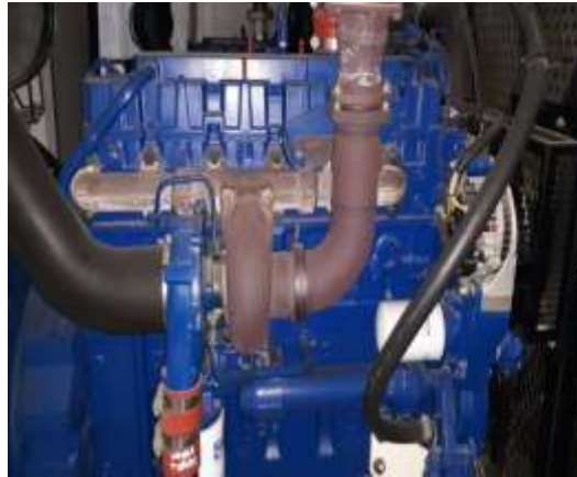
Fig. 2. Turbocharger System
