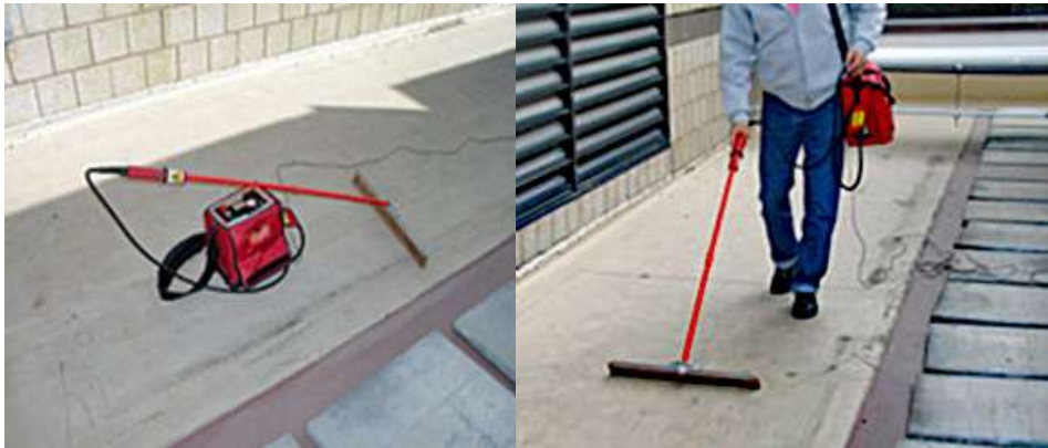
Figure 6.High voltage test equipment
