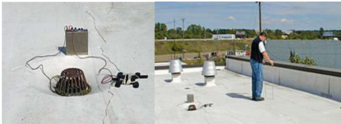
Figure 2. Low voltage test equipment
