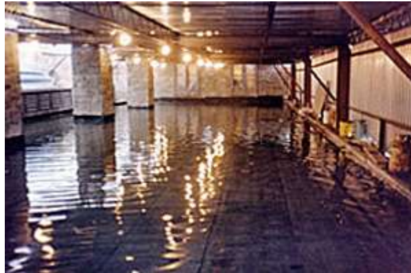
Figure 7. Flood testing in progress
