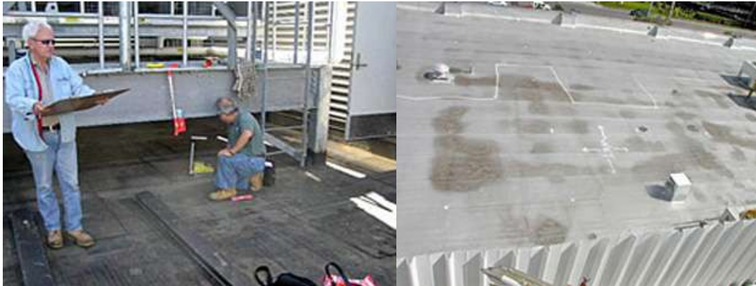
Figure 11. Nuclear meter (yellow) and grid pattern on roof
