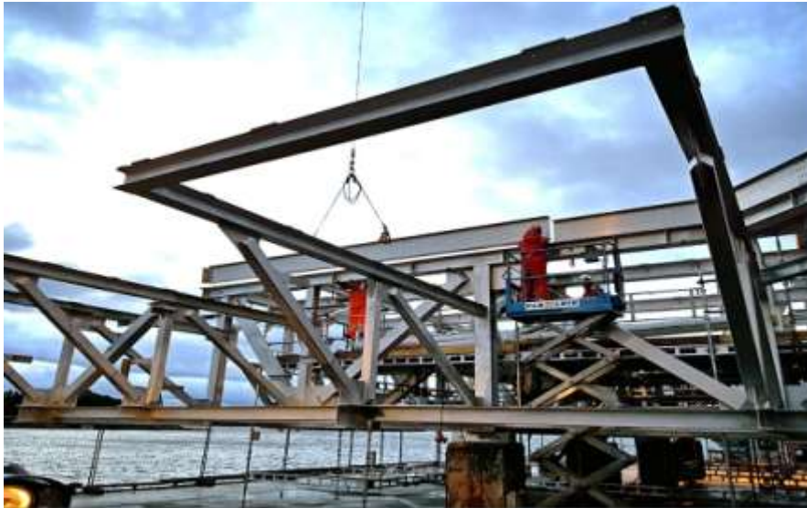
Figure 3: Pictorial View of a Helideck trusses Sourced:(Offshore, 2015)
