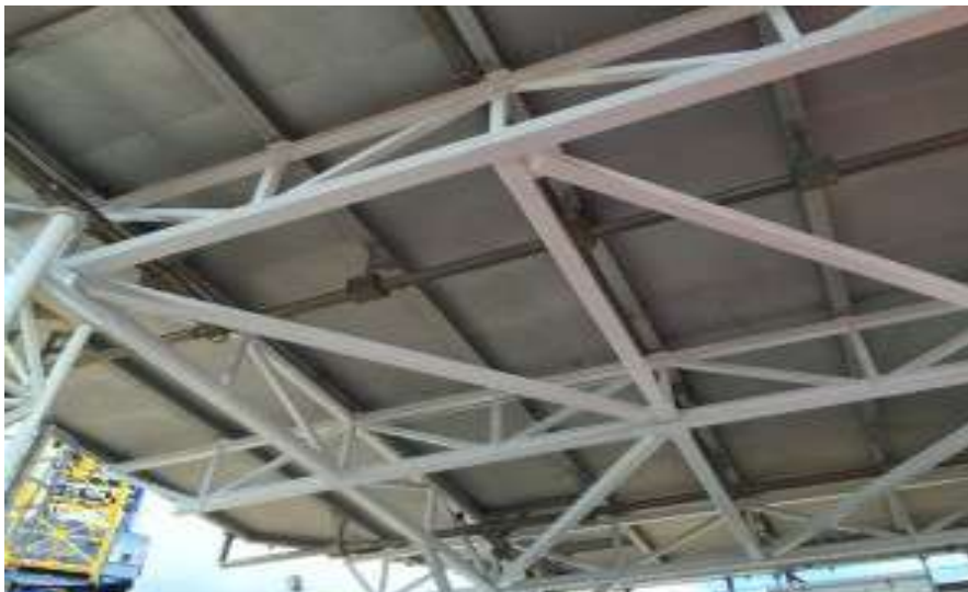
Figure 4: Pictorial View of a Helideck frames Source:(abfad, 2014)
