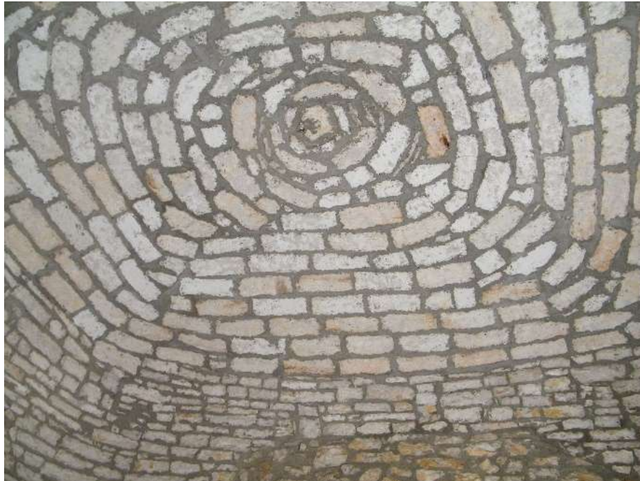
Fig.13. Semi-spherical vault of tuffaceous stone
