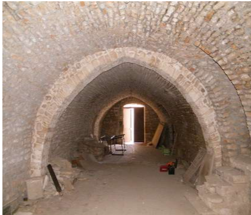
Fig.11. Vault of limestone
