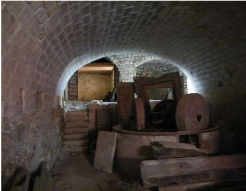
Fig.9. Vault of tuffaceous stone
