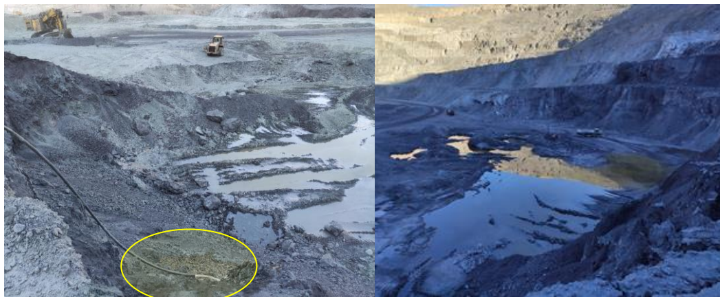
Figure 8. Unsuitable Dewatering and Wall Saturation Condition in Downstream of New Dangerous Area (Winter)
