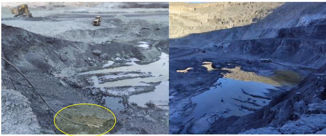
Figure 8. Unsuitable Dewatering and Wall Saturation Condition in Downstream of New Dangerous Area (Winter)
