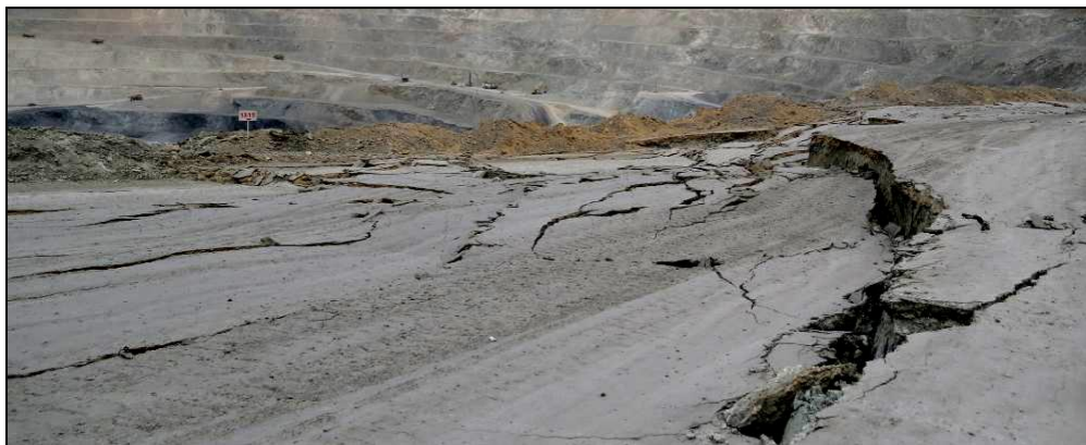
Figure 13. Adaptation of the main crack direction with faults direction in the unstable area and the destructive effect of groundwater on the strenght parameters of the gouges.
