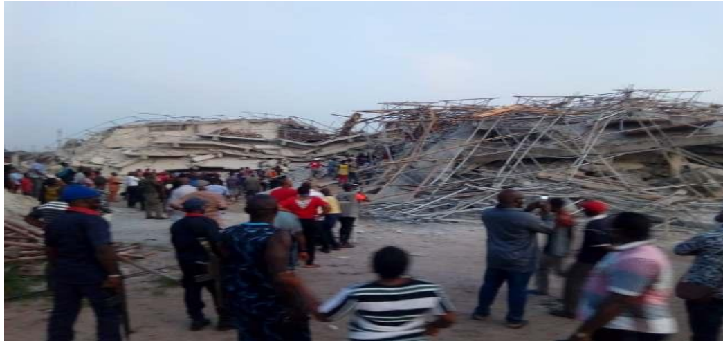
Fig. 1: 2020 Owerri building collapse [5]
