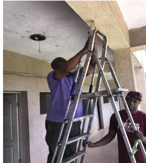
Fig. 8: Field investigation on a beam
