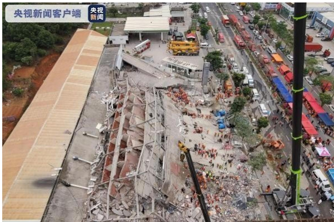
Fig. 2: 2020 Xinjia express hotel Collapse [12]
