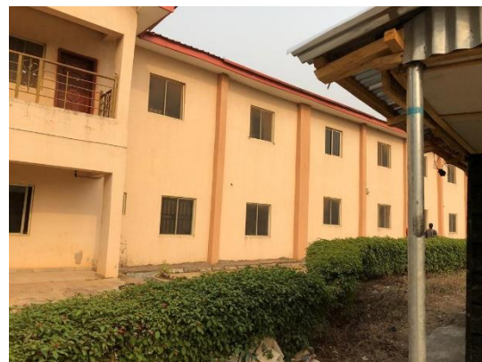
Fig. 6: View of Hostel B
