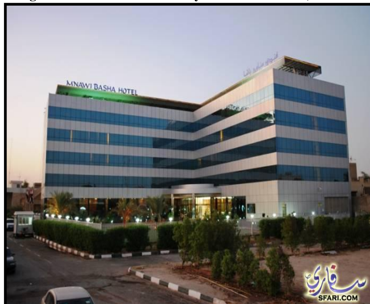
Fig.2. Modern Architecture in Basra City (Mnawi Basha Hotel)
